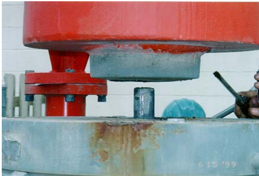
Figure D-9 Tower jacked up to approximately 1/2-inch above center pin of base insulator.
