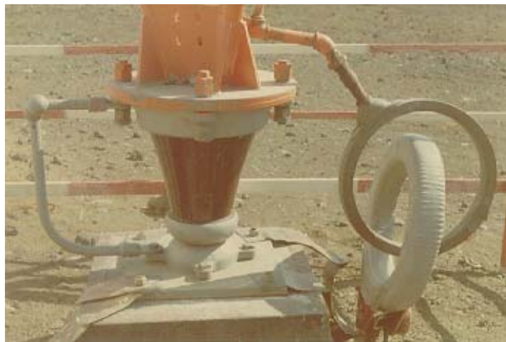
Figure 5-3 Cone shaped base insulator.
