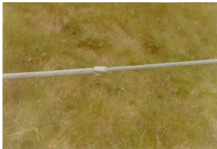
Figure 6-3 End sleeve installed on guy-grip dead end.
