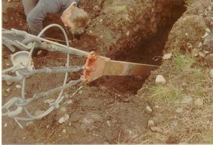
Figure 4-1 Excavation and inspection around anchor arm.
