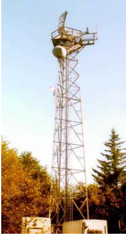
Figure 1-2 90ft Self supporting Vessel Traffic System tower.
