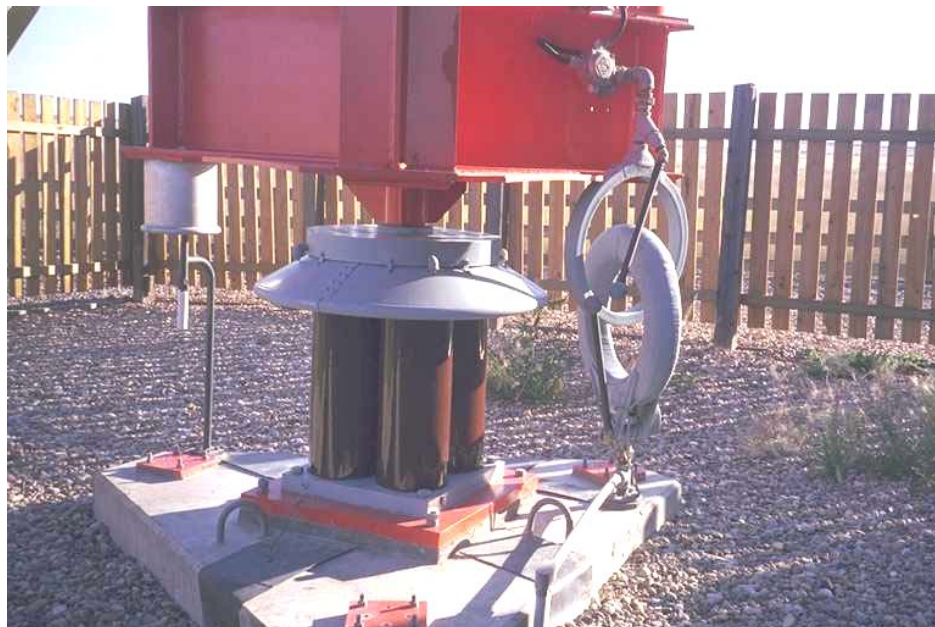
Figure 5-6 Oil-filled multiple cylinder base insulator.
