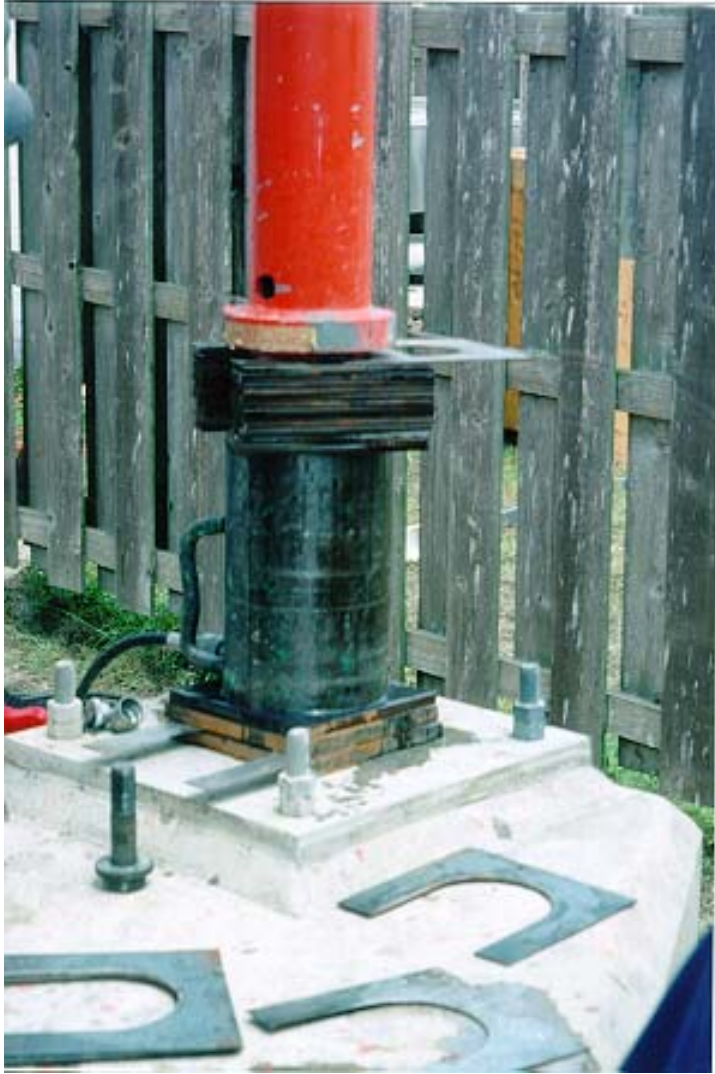
Figure D-7 Shims between jack and tower jacking leg.
