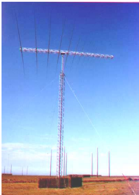
Figure 1-5 Guyed rotatable antenna
