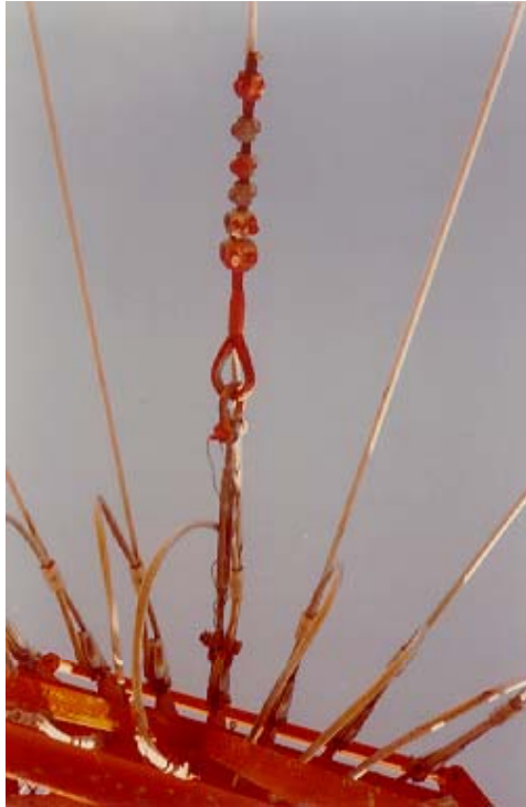
Figure 6-4 "Sister Wire" consisting of shackles, turnbuckles, wire rope segment with preformed eye, reinforcing a TLE on a Loran tower.
